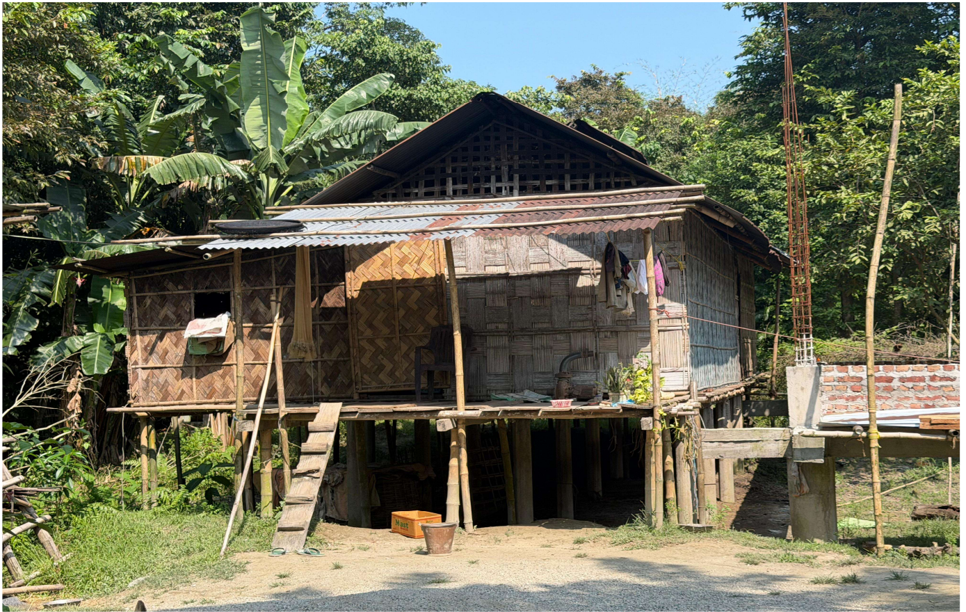
A representative Deori Chang Ghar stilt house showcasing traditional settlement layouts and community-centric vernacular architecture in rural Assam
